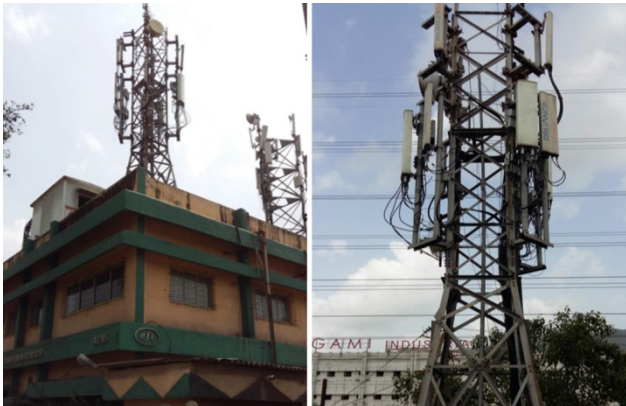
Figure 1. Upgrading a cell tower with FTTH
